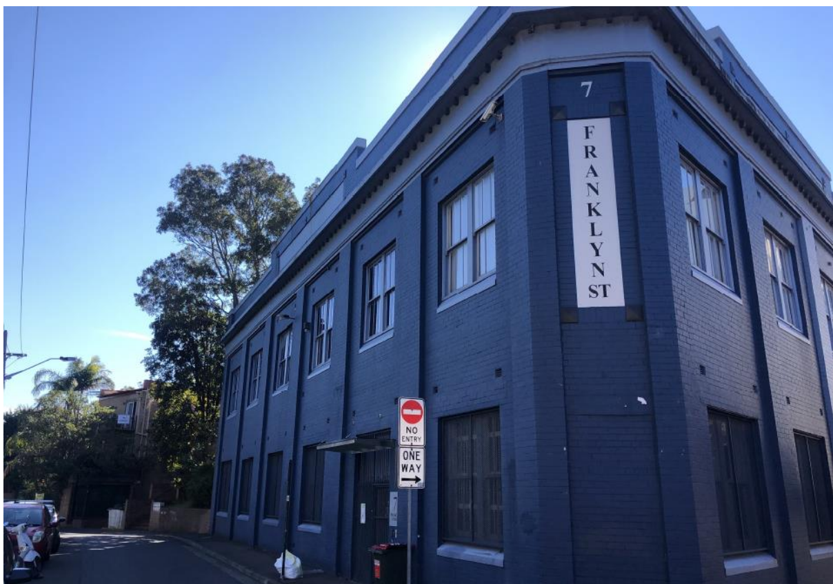
Figure 2: Site viewed from corner of Franklyn and Greek Street (building shown is 7 Franklyn Street)
