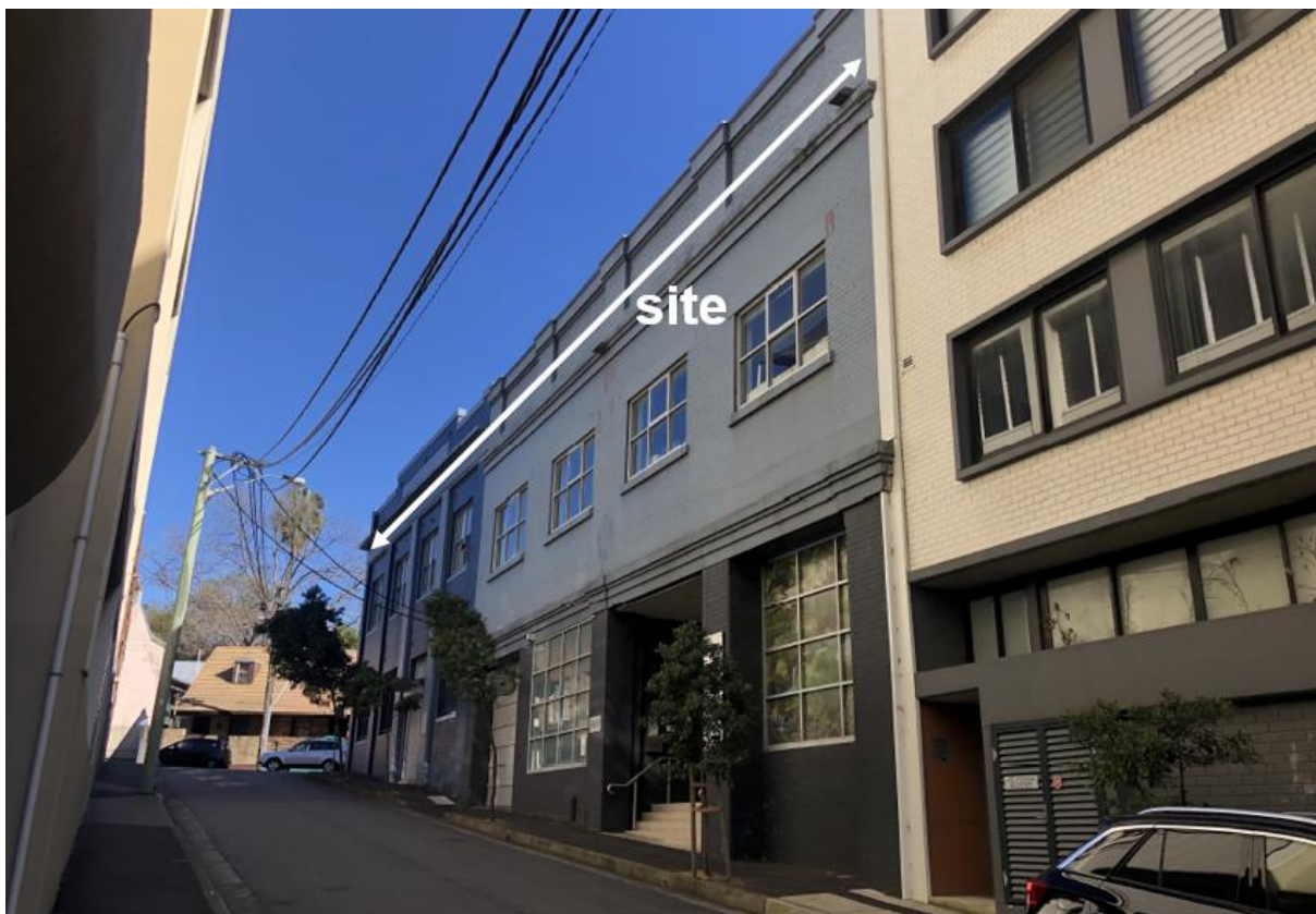
Figure 4: View of site looking west up Greek Street (49 Greek Street shown in foreground)
